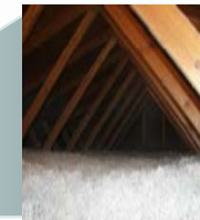
Increased attic insulation (R30-R38)
